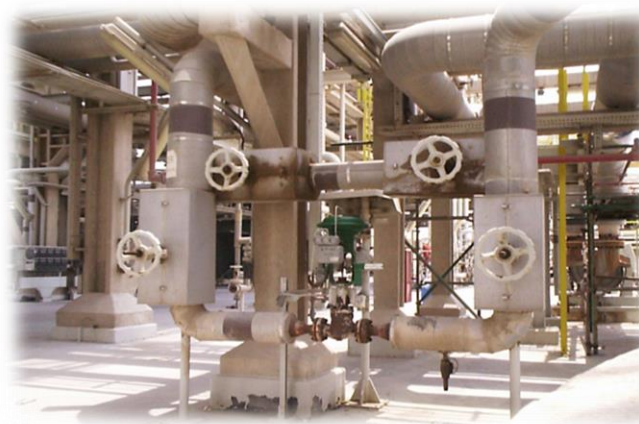
CHESTERTON 5150 VALVE LIVE LOADING system used to eliminate leakage and prevent emissions of hazardous gases at critical valves.
