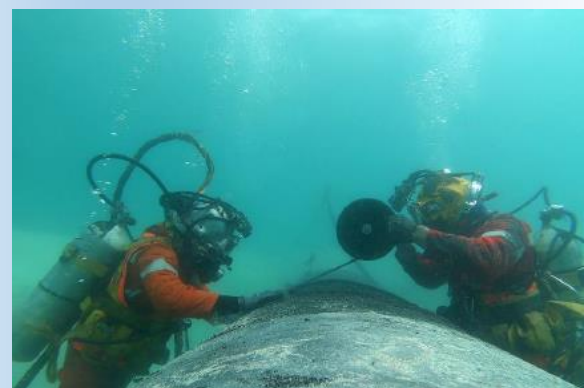
Figure 3: Composite wrapping on progress (step 5)
