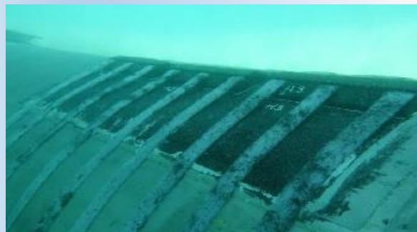
Figure 2: Composite plate application using F3XSS filler and ratchets belts (step 3)
