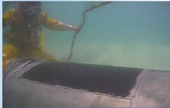
Figure 1: P3X30 primer application on defected area (step 2)
