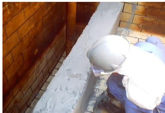
Applying of ARC 791 by Chesterton specialist
