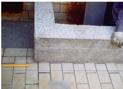
Wall after surface Preparation and decontamination
