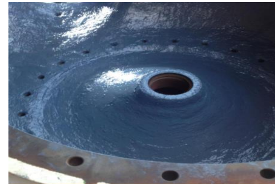
After application of ARC BX1 and ARC S2
