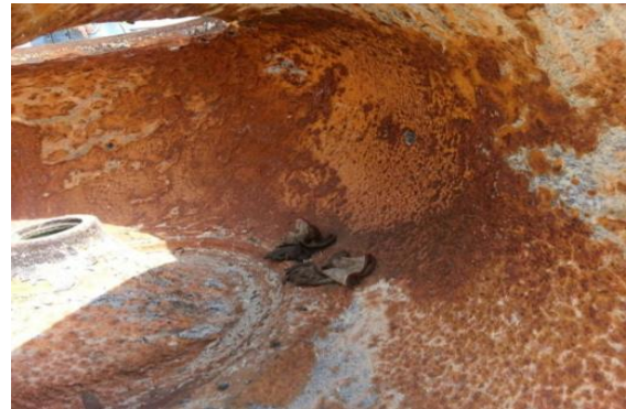
Worn pump before application of ARC BX1 and ARC S2
